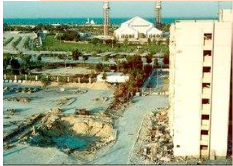
Khobar Towers, Saudi Arabia, Jun 25, 1996: The building did not suffer progressive collapse in spite of the massive bomb blast which left a large crater in the ground.
