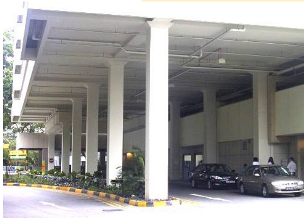
Columns near vehicular traffic.
