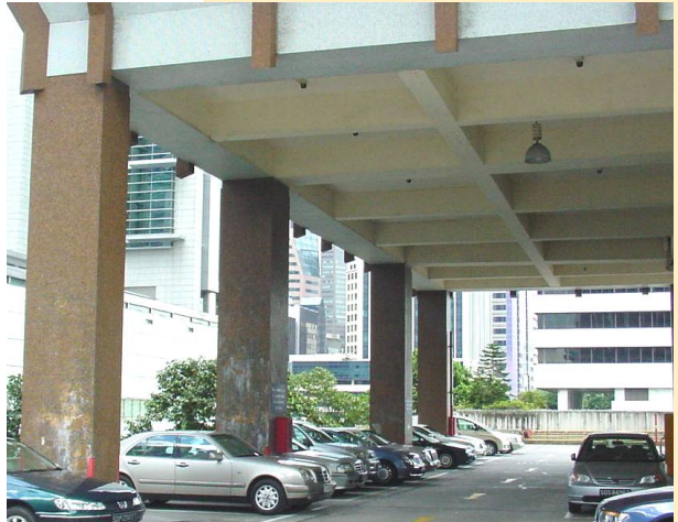
Transfer beams above a car park.
