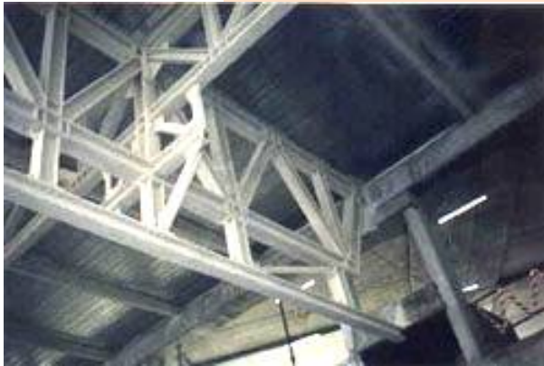
Examples of fireproofing for structural steel.
