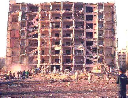
Khobar Towers, Saudi Arabia, Jun 25, 1996: The building did not suffer progressive collapse in spite of the massive bomb blast which left a large crater in the ground.
