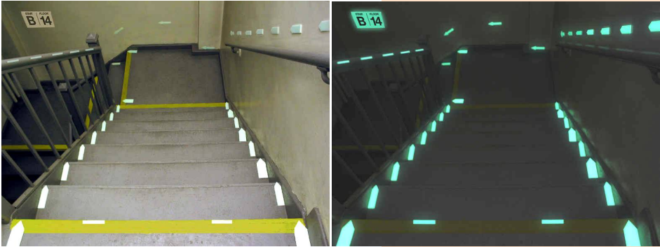
Provision of self luminescent markings along a staircase.
