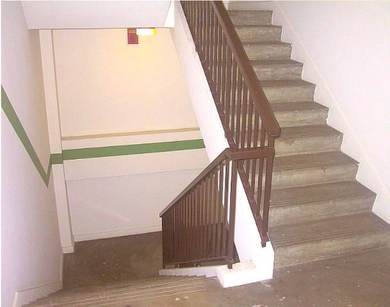
Reinforced concrete staircase cores.
